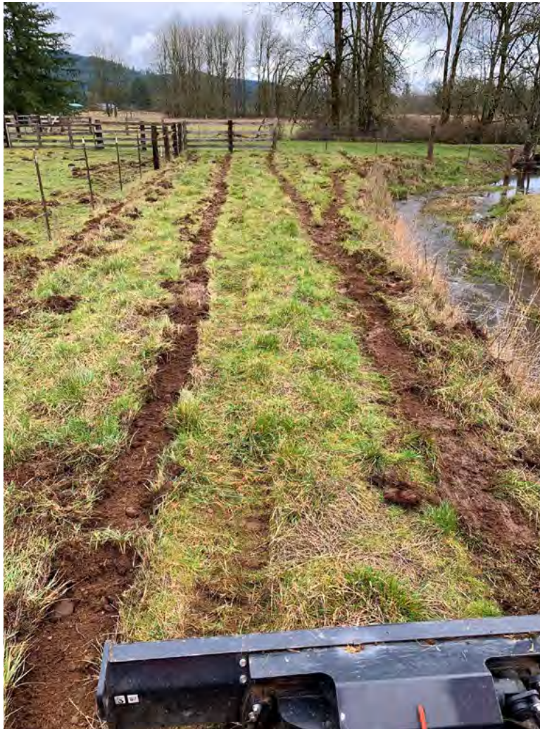
▲ Site prep for this hedgerow utilized on-farm equipment to quickly remove pasture grasses from the planting area, with a maintenance plant to mow the grasses between the rows until the hedgerow matured enough to shade out or displace them. A sod pile from this type of prep can be sheet mulched, creating a compost-rich planting soil within a year or so after the smothered grasses have decomposed. (Photo: Kevin Jensen)
