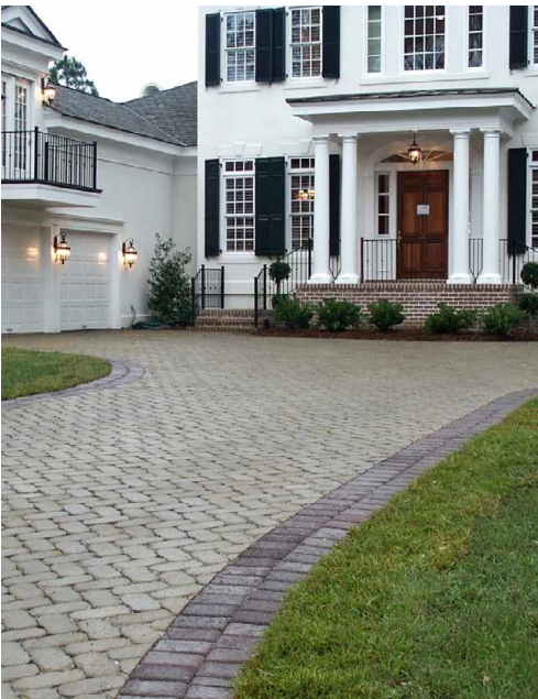
Pervious pavers filter and manage water on site. Photo: Interlocking Concrete Paving Institute.
