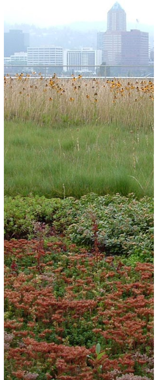
Green roof, Portland, OR. Photo: Erica Guttman
