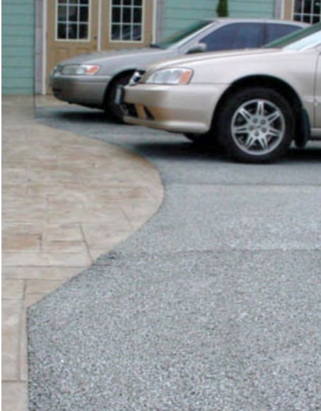
Ribbon driveway, steppable plants with stones, permeable concrete & permeable pavement. Photos: Erica Guttman, Curtis Hinman, Interlocking Concrete Paving Institute
